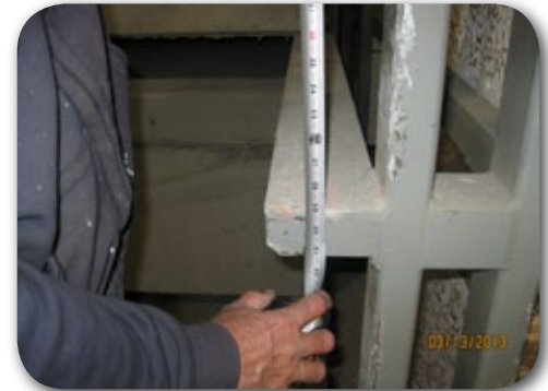
Custom built vault racks average measured height allowance
