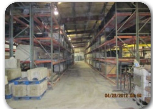
Converted racks from Home Depot®
